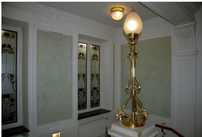
7. Replicas of colored acid etched glass panel in staircase made in Nový Bor, Czech Republic (photo: Marija Režek Kambič, ZVKDS, OE Ljubljana)
