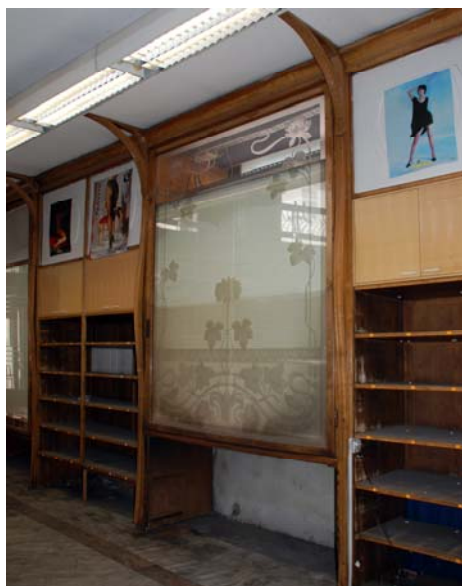
9. Acid etched glass panel in 2009 (photo: Marija Režek Kambič, ZVKDS, OE Ljubljana)
