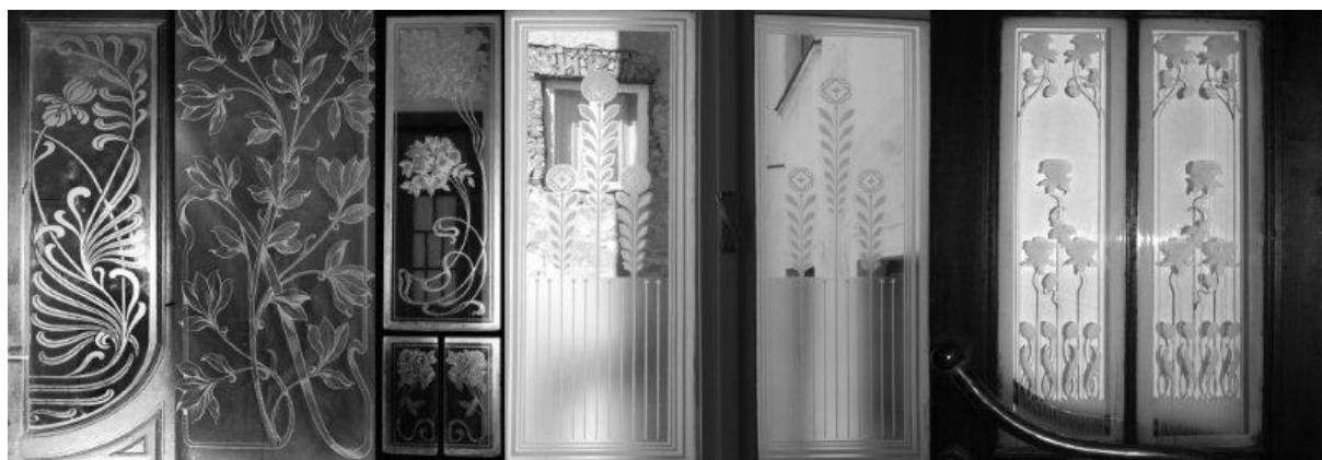
4. Acid etched glass panel with Art nouveau motifs (photo: Marija Režek Kambič, ZVKDS, OE Ljubljana, photo: Carmen Narobé, documentation MGML)
