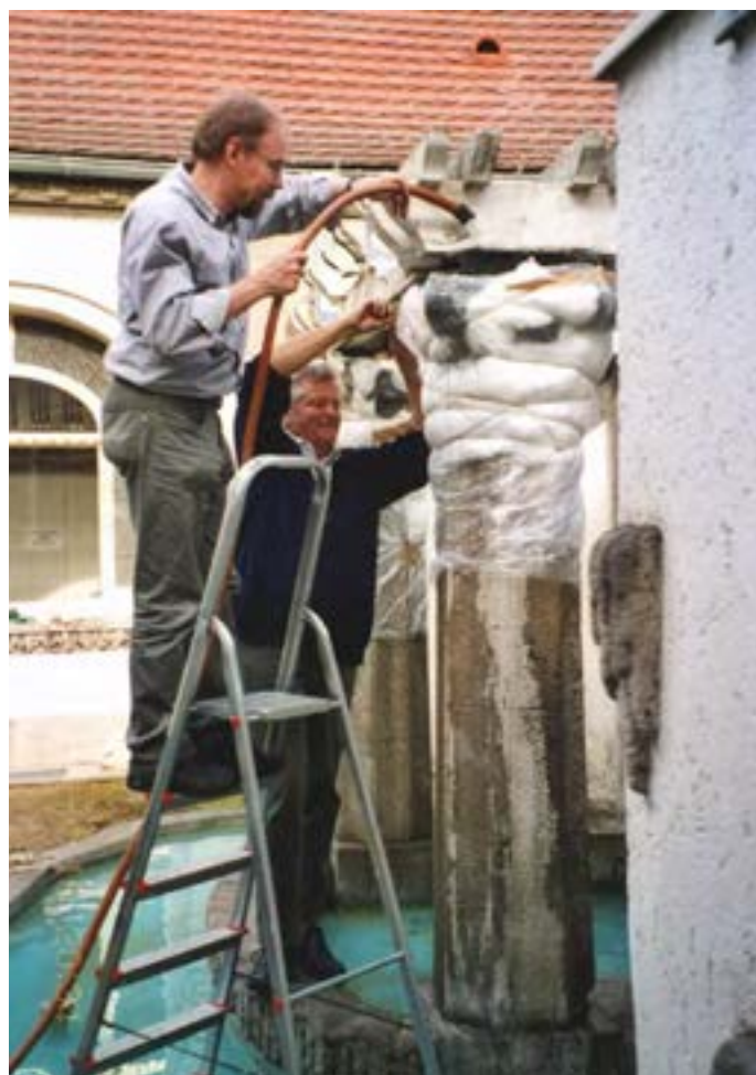
Figure 4: bath house 5, restoring the fountain
