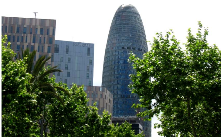
Agbar Tower (photo: Saida Palou)
